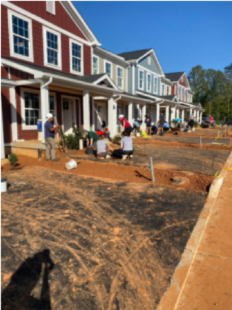
Volunteers landscaping 8 townhomes. Photo: M Costanzo
