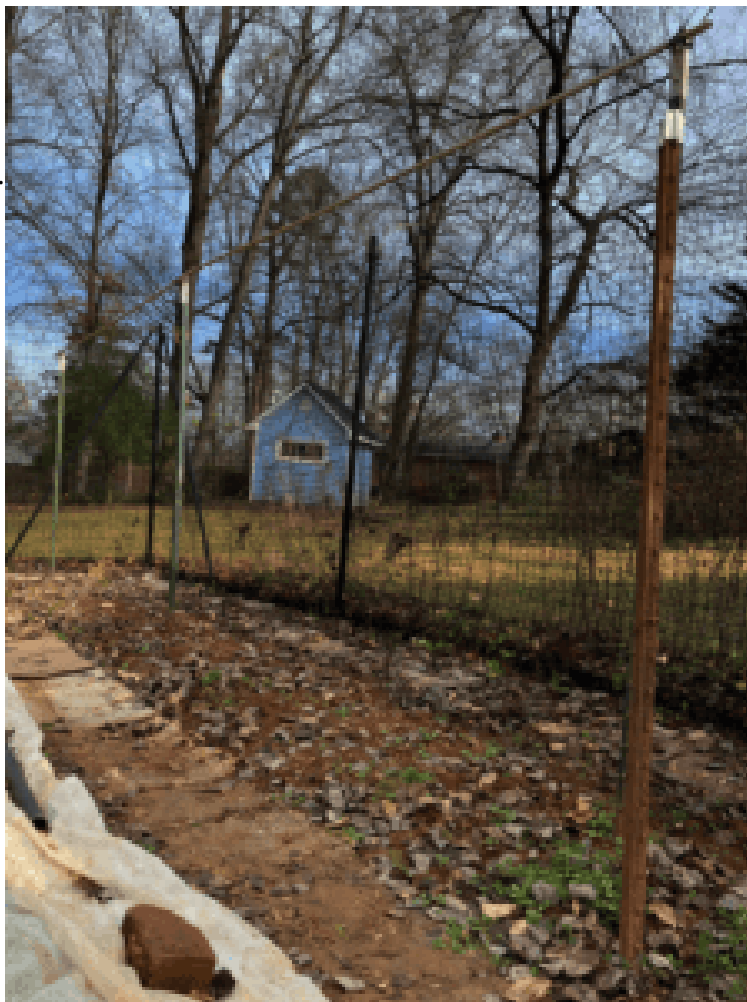
Make an overhead support by running conduit down the row, supported by fence posts. Image: © 2022 S. Christopher Stroupe
