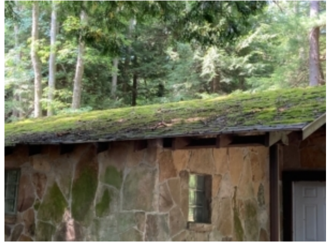
Moss growing on rooftop in shady spot in the woods; photo: Melissa King
