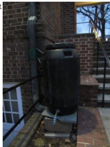
A plastic tank collects water from a downspout for use in a courtyard. Photo: David Garth
