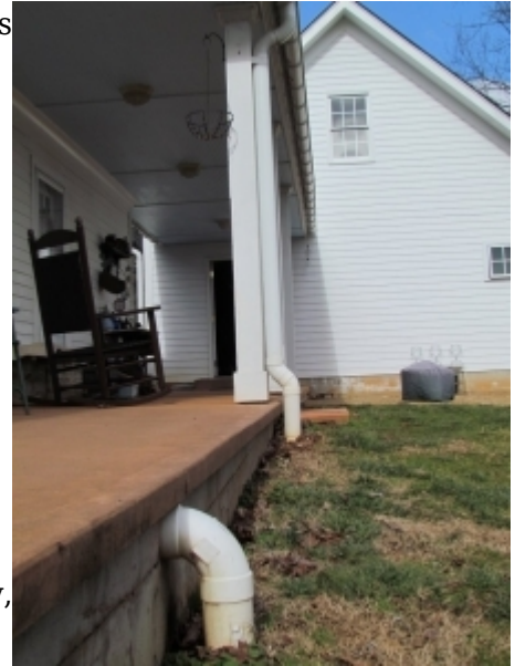
Water from the gutters goes underground to a 2400 gallon cistern. Photo: David Garth
